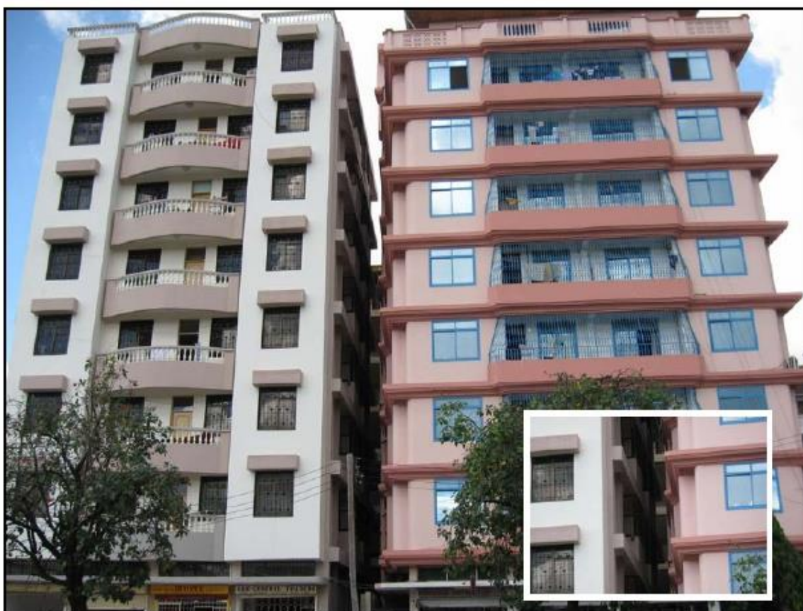
Photo 5: Two buildings with blocked lighting and ventilation: the case of T-4 and T-5, located along Lumumba Street (Source: Based on fieldwork studies in Kariakoo area, March 2008).
