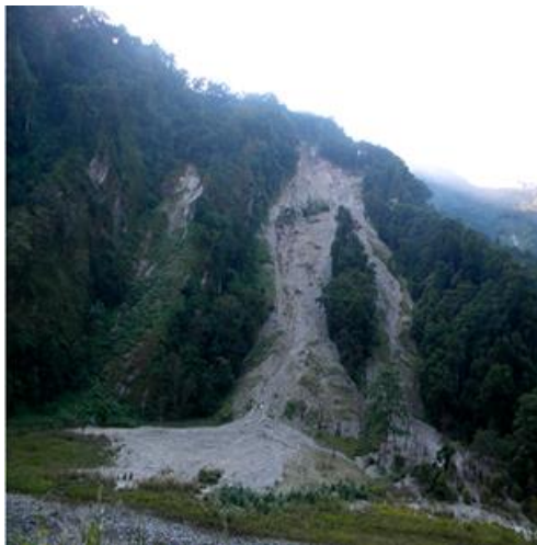
Plate-8: Debris Fall near Pankhabari
