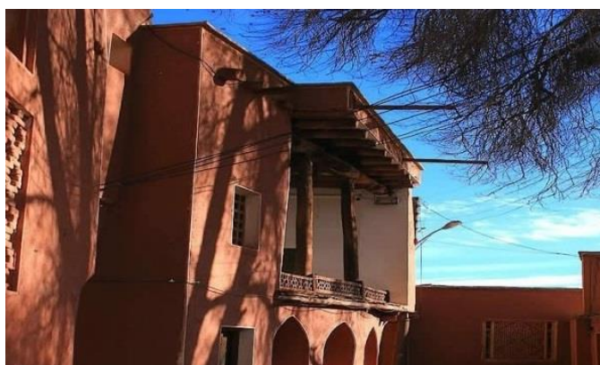
Fig-3: building in abyaneh
