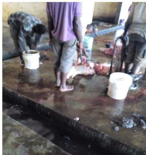
Fig-2: Slaughtering and Butchering on unkempt floor of the slaughter hall
