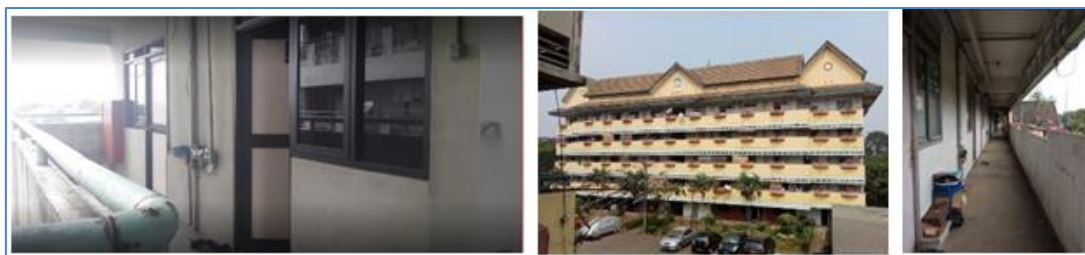
Fig-1: Condition of rental apartments
