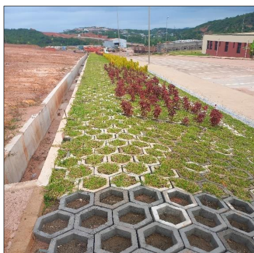
Figure 3: Overview of a semi-vegetated surface showing cells being revegetated
