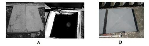
Fig. 1: Water storage tanks before the cleaning procedure (A) and after washing and exchanging of lids (B)
