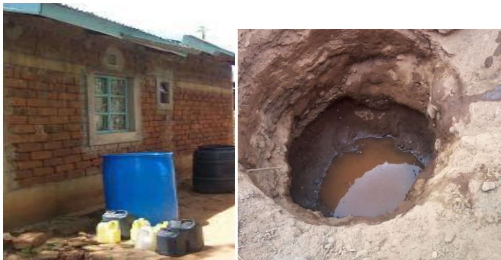
(a) Jerry can storage facilities in Salabani (d) Dug well in Ribkwo Plate 1: Various Rooftop Rainwater storage Facilities used in Baringo County. Source: Field data, August 2015
