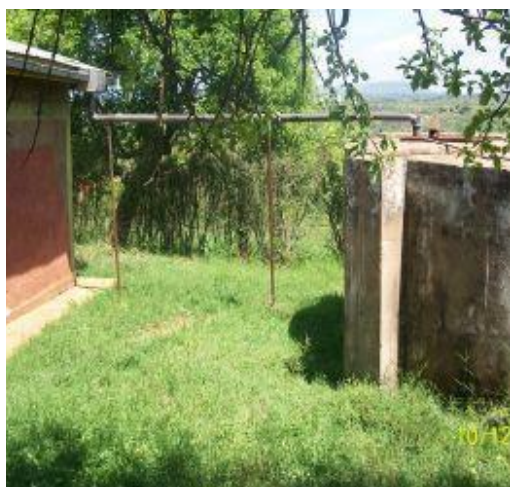
(a) Cement tank in Lembus Central
