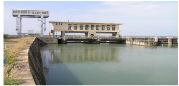
Ph 11: Main vue of the Lagdo Dam, MINEPIA, 2008 Source: MINEPIA 2014 [22].
