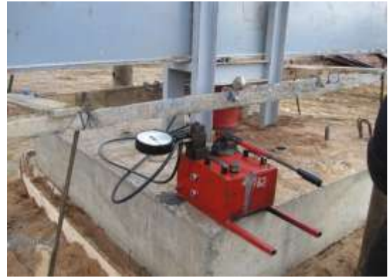
Fig.3: Hydraulic jack for field test loading
