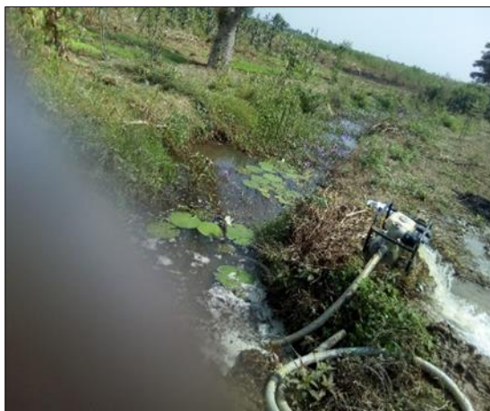
Figure 3 : Dewatering with the motor pump
