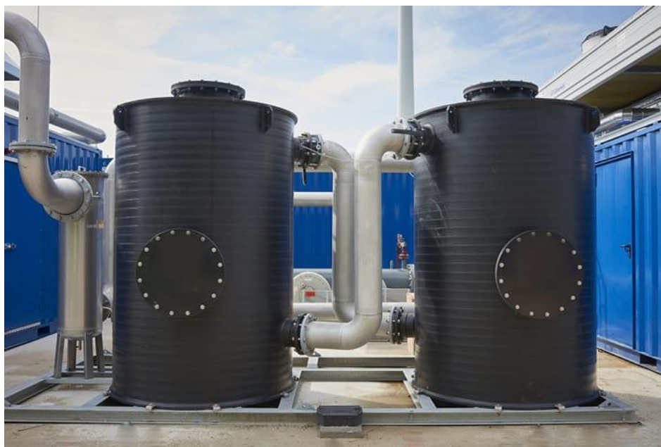
Figure 10: Biogas scrubbers desulfurization
