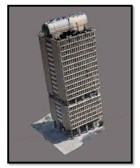
Fig-7: The Dense point cloud of UOB Tower
